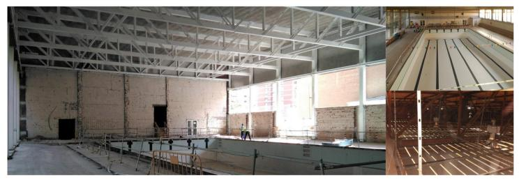
The building intended for indoor pool and pavilion has a height of approximately 23.20 m, with plant dimensions of approximately 62x25 m.
